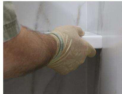
Avoid large gaps between the Wetwall surface and corner shelf by sanding, or cutting to ensure good fit to wall panels.
