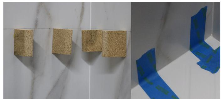
Place a piece of blue painters tape on top of support block, so that sealant does not prevent removal of support blocks after cured.
