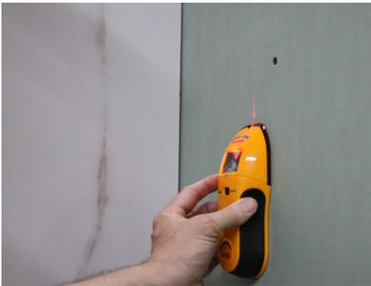
Determine location of recessed niche (Standard height for the recessed shelf would be 43" from the shower floor to the bottom of the opening).
