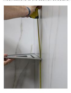
Using a level, mark location where corner shelf is to be installed on the Wetwall panels. (Recommend the Corner Shelf would be installed 43" from the shower floor).
