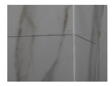
Dry fit corner shelf to ensure good fit to wall panels, so that you do not have large gaps between Corner Shelf and panels.
