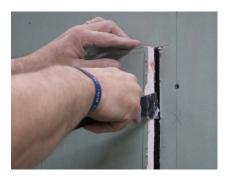
Cut and remove the current substrate (tile, green board, cement board) to expose the wall structural framing.
